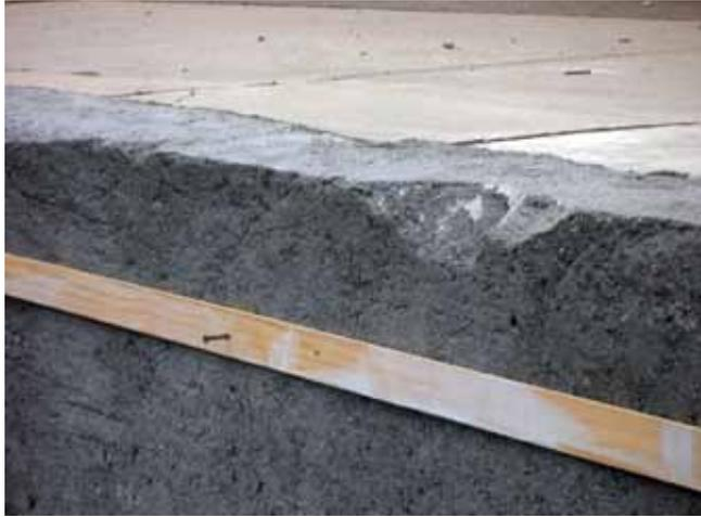
*Batter board attached to the pool shell with concrete nails. Note the minor damage to the top of the pool wall*
