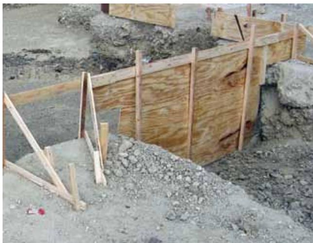
*After shotcrete, backfilling of the pool wall will be necessary before work on the pool can continue*
