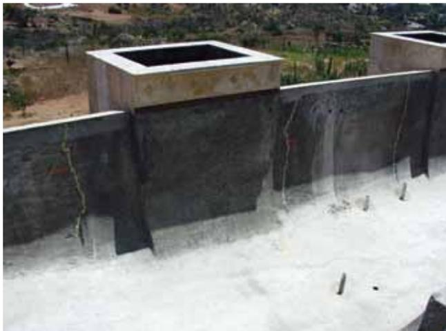
*Vanishing edge weir wall where shrinkage cracks reflected through water line tile. Repair was by epoxy injection*
