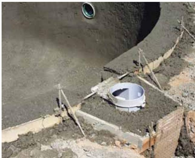
*Typical bender board form work around a swimming pool that sets the shape, elevation, and dimensions*
