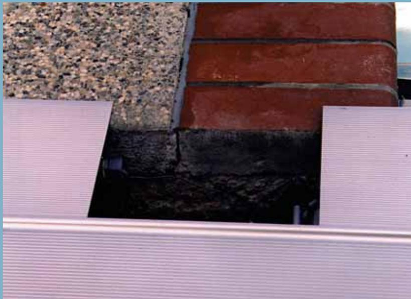
***Here's a caution: In some situations, tamping can force decking concrete beneath a mastic joint, thereby negating that joint's benefits. In this case, the lifting of the deck yanked the coping out of its bed; shortly after this photo was taken, some of the coping stones broke free!***
