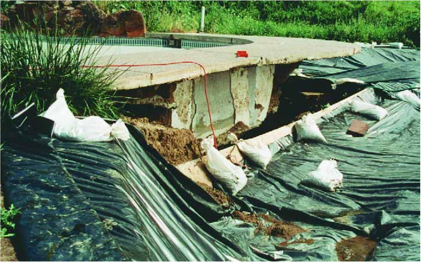
**THE BUILDER'S** lack of awareness of the unsuitability of this soil resulted in a classic case of differential settlement – in this instance, one that had a devastating effect on the decking at one end of the pool.
