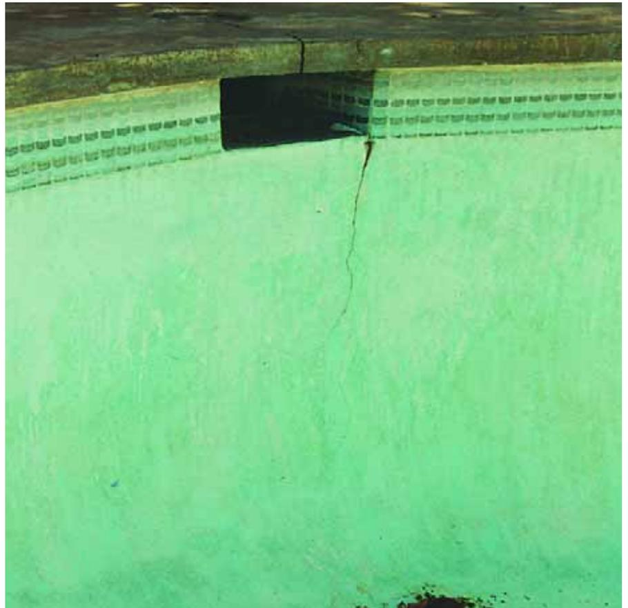
**IT'S NOT ALWAYS** the case, but very often the kind of cracking that appears around skimmers has as much to do with a failure to observe basic building codes as it does with the hinge effect and differential settlement. The skimmer is the shell's weakest point and must be engineered and installed properly.
