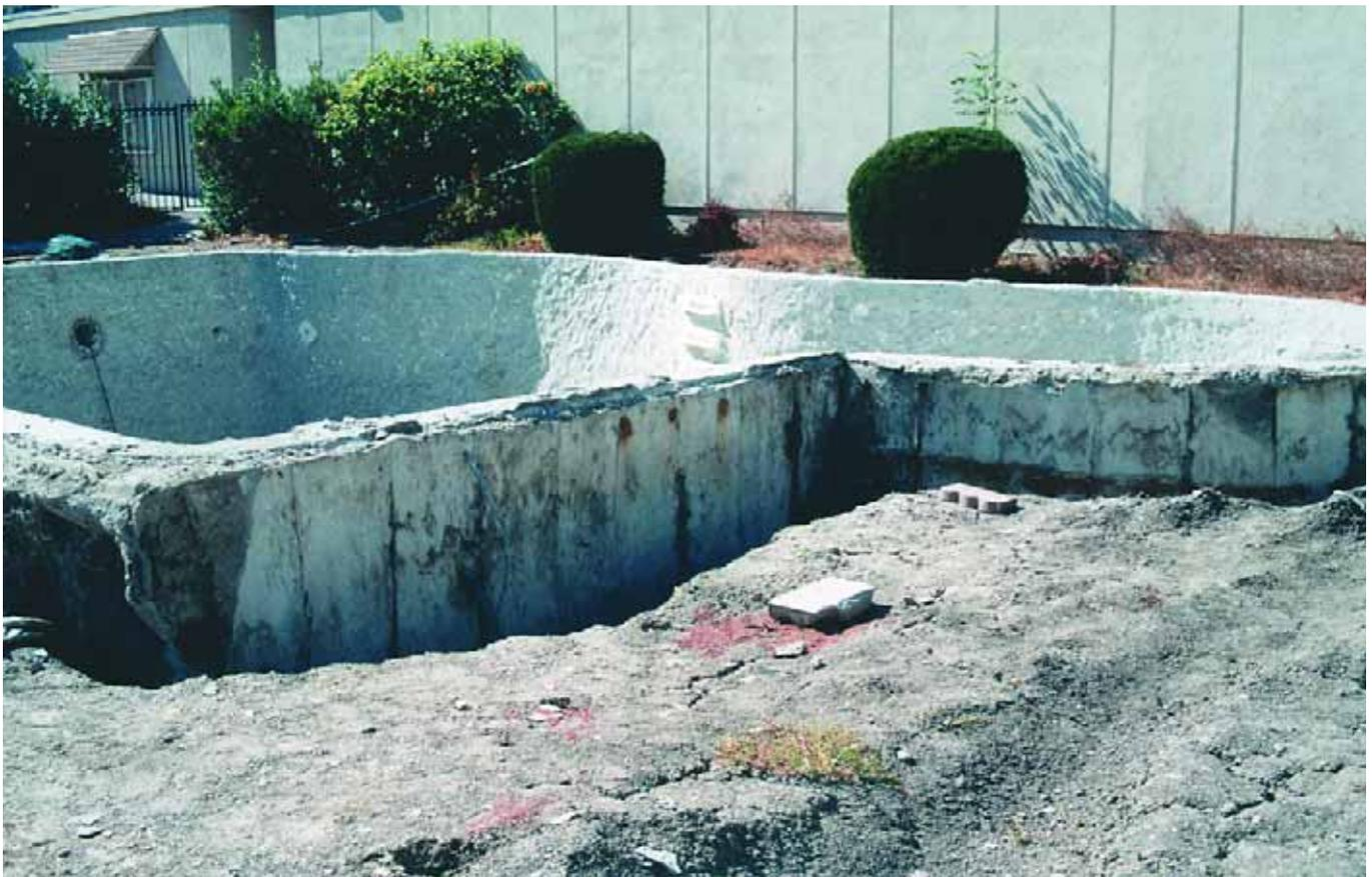
**ONCE THIS POOL** had been emptied of water as part of a renovation, the water in the surrounding soil caused the shell to float up and literally 'pop' out of the ground – testimony to the amazing subsurface pressures that sometimes impose themselves on concrete shells.
