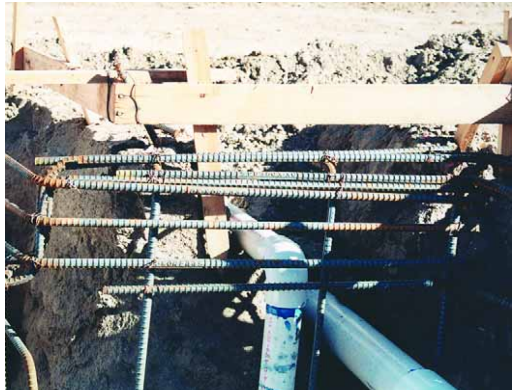
Steel does a fantastic job of reinforcing when it is set up and tied to allow for proper pneumatic application of concrete. In these two cases, however, steel's ability is severely compromised by improper lapping that very often results in the creation of voids as the concrete is applied.
