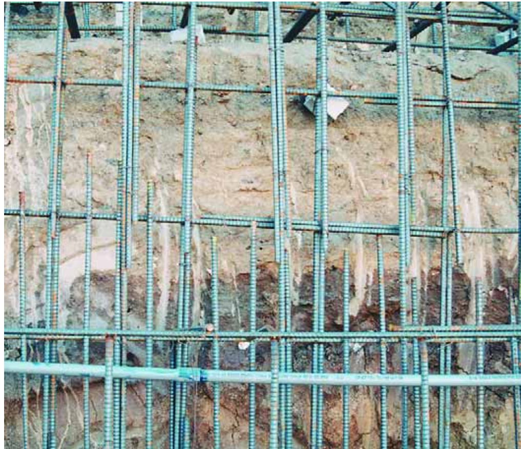
Steel does a fantastic job of reinforcing when it is set up and tied to allow for proper pneumatic application of concrete. In these two cases, however, steel's ability is severely compromised by improper lapping that very often results in the creation of voids as the concrete is applied.
