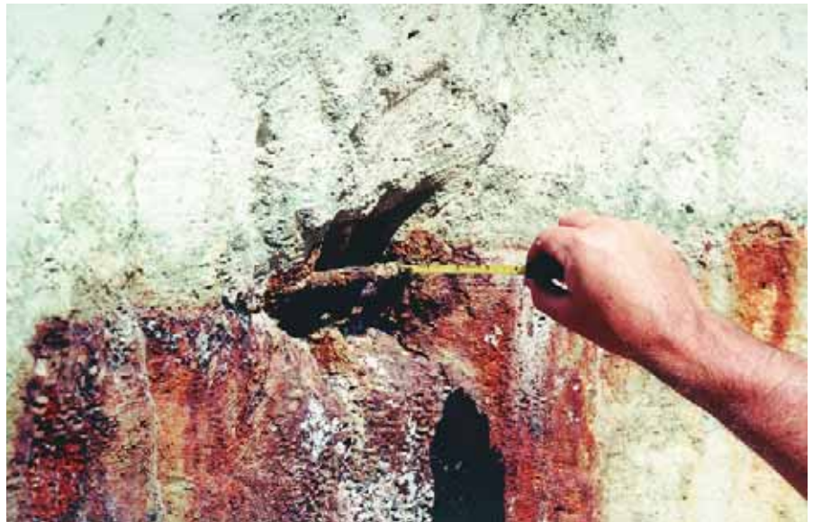
It is extremely important to encase reinforcing steel in adequately thick layers of concrete. As the photo that opens this article shows (page 54), steel set in shallow concrete will fail in dramatic ways. When such vessels are stripped for repairs, the true extent of the disaster is plainly seen.
