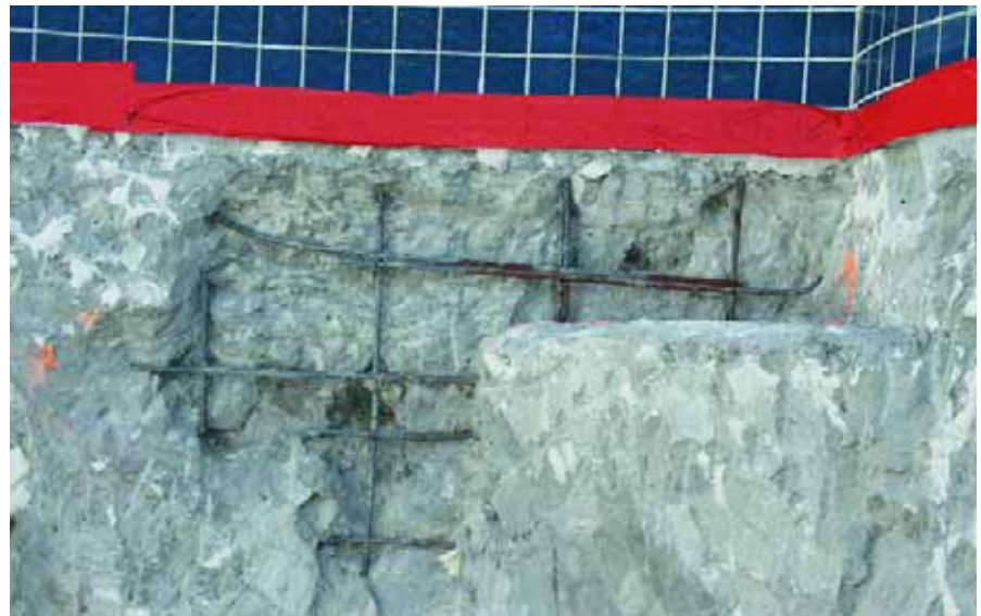
It is extremely important to encase reinforcing steel in adequately thick layers of concrete. As the photo that opens this article shows (page 54), steel set in shallow concrete will fail in dramatic ways. When such vessels are stripped for repairs, the true extent of the disaster is plainly seen.
