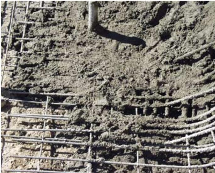
*This trimmed material sat in a pile at the base of the wall for over 90 minutes. Remember, concrete consolidation and reinforcement encapsulation are critical elements of structural concrete placement*
