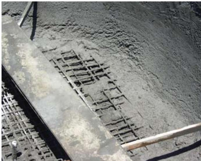
*The trimmed concrete typically lands at the base of the wall on top of rebound and overspray*
