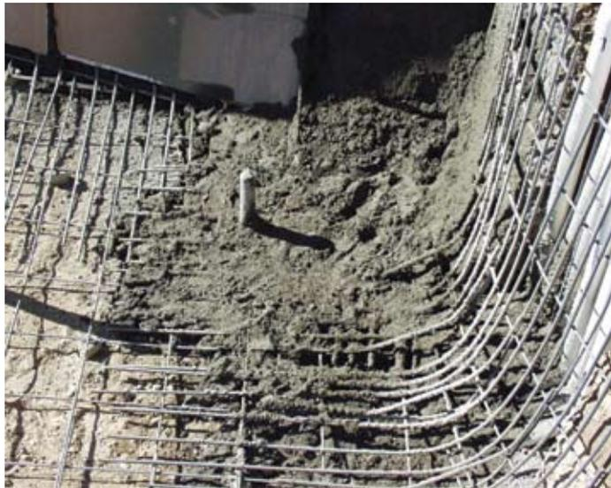
*Trimmed shotcrete is no longer consolidated after falling from its shot location and landing on the pool floor*
