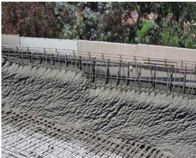
*In swimming pool wet-mix shotcrete application, it is common practice to shoot the pool walls first while leaving the floor at the base of the wall open. Note the overspray, rebound, and voids under the reinforcing bar*
