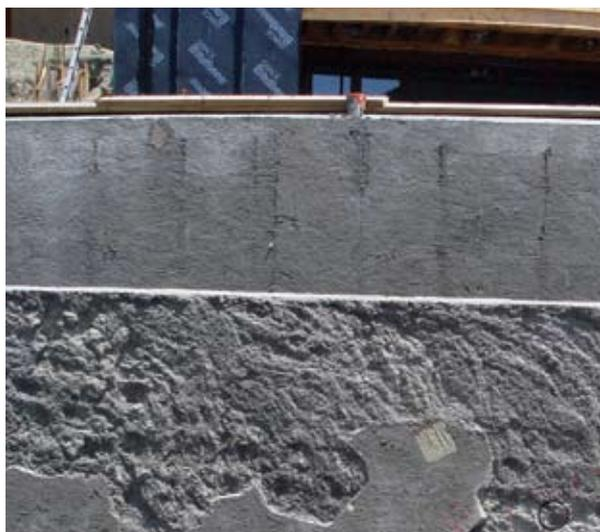
*When the forms were stripped, the outer surface of the basin wall delaminated, leaving substandard coverage over the reinforcement. Note the exposed reinforcement in the weir wall in the background*
