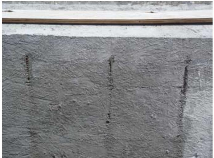
The dobies slipped out during shotcrete application, allowing the reinforcement and formwork to come together, leaving essentially no cover over the reinforcement
