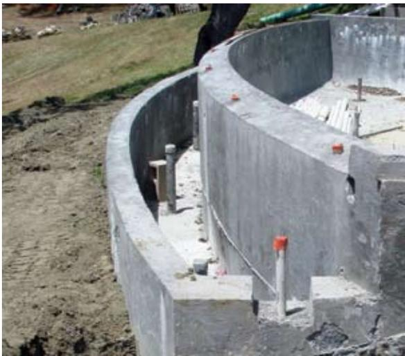
On vanishing edge pools, the weir wall and often the outer basin wall must be formed for shotcrete application. Forms are usually erected on the outside of the wall
