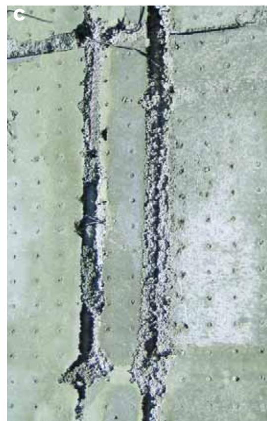
Workmanship plays a definite role in these problems with weir walls. Situations in which cages are inadequately secured and are able to move during shotcrete application are trouble (A), for example, as are instances in which no spacers are used to make certain rebar can be fully and completely encapsulated in concrete (B). The consequences in the latter case show up as soon as the forms are stripped (C) – and the situation only gets worse when water is introduced.
