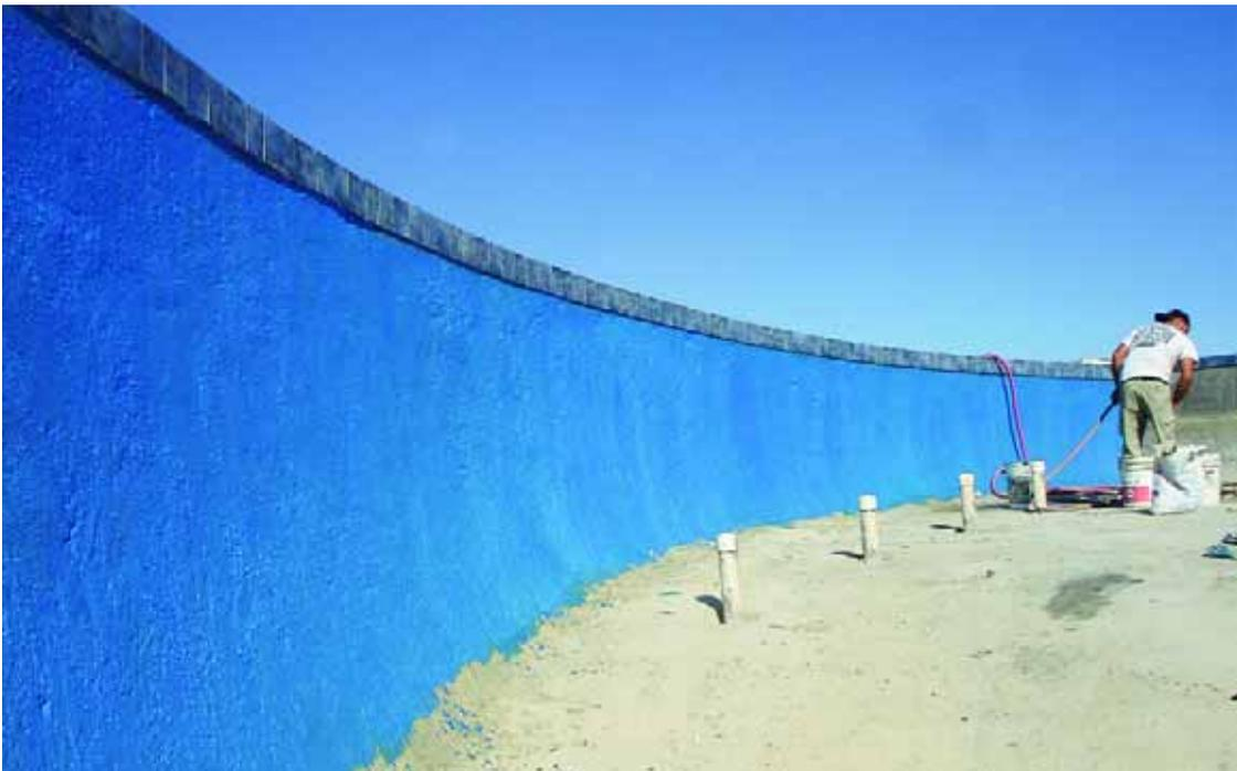
Waterproofing is a good idea on both sides of a vanishing-edge weir wall, simply because, when properly applied according to manufacturer instructions, these coatings minimize the transfer of water from the pool to the outside of the wall and thereby act as welcome layers of protection.
