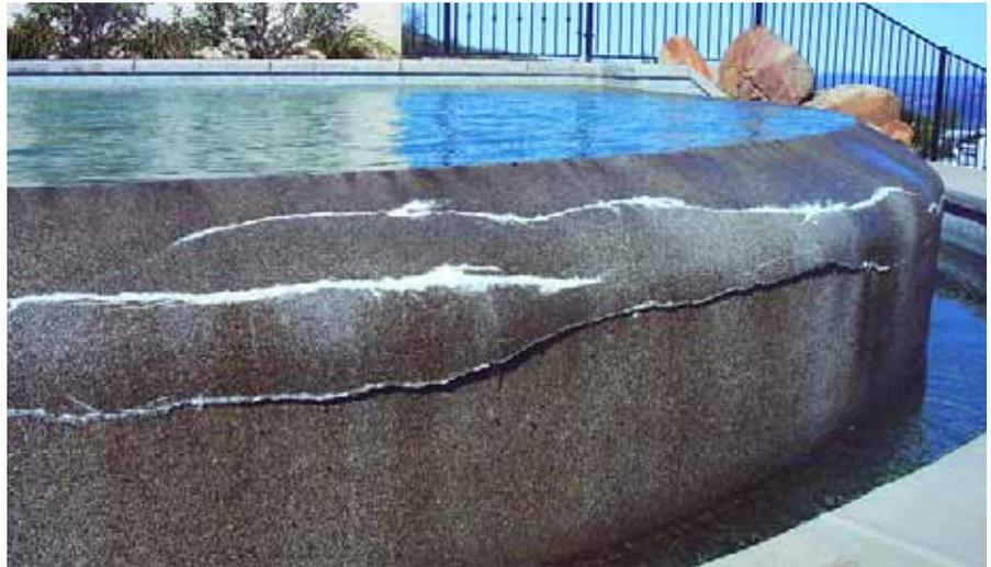
In the years since vanishing-edge pools gained incandescent popularity in the 1990s, we've seen more and more failures of the sorts depicted here, with extensive, disastrous cracking and delamination of surface materials. It took a while, but eventually patterns emerged that helped us determine why these freestanding weir walls were failing – and what needed to be done to prevent it.
