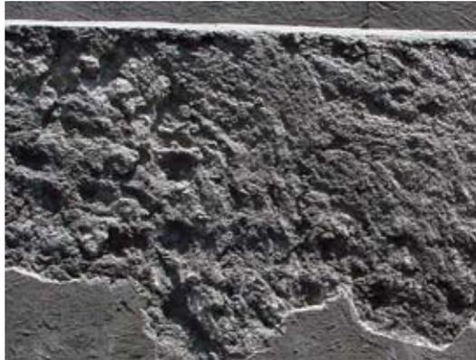
*Fig. 9: After the forms are stripped, this becomes the receiving surface for shotcrete on the alternate side. Results in questionable bond and reinforcing bar encapsulation*
