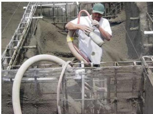
*Fig. 4: Another questionable practice: an expanded metal lath is tied directly to the reinforcement and left in place between the inner and outer layer of shotcrete*
