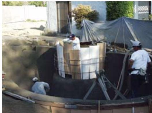
*Fig. 5: Unacceptable practice: drywall form held directly against reinforcement by crew member without dobies or spacers to establish the cover over the reinforcement*
