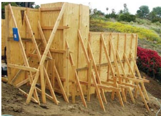
*Fig. 3: The most difficult and complex forming is required when a swimming pool is built either partially or completely out of grade*
