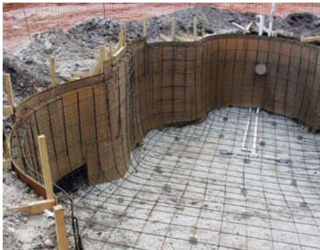
*Fig. 2: In Florida and several areas of the northeastern U.S., the perimeter of swimming pools is often over-excavated then usually formed using steel-tex, a paperback wire mesh*
