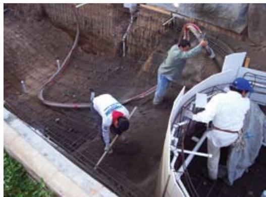
*Fig. 6: Drywall form often placed on the outside of the reinforcement and the wall shot from the inside. Only tie wire on the outer face is holding the drywall in place*
