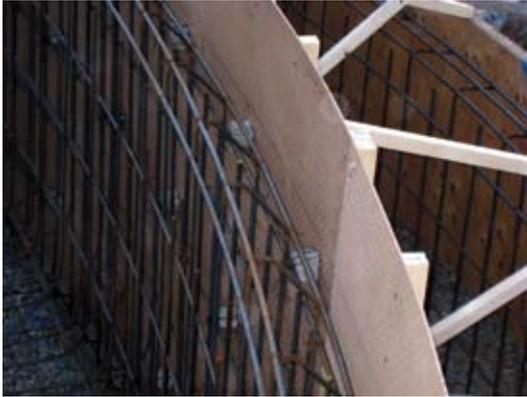
*Fig. 7: Example of secure dam wall forming braced to resist vibration and the impact force of the shotcrete. Reinforcement tied to forms with dobies to resist vibration and provide proper coverage*
