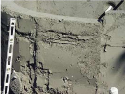
*Fig. 8: Delamination occurred when forms were stripped. The surface against the form contained sand lenses and trapped overspray and rebound*
