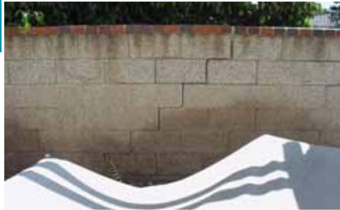
**Side property line walls will crack usually 10 to 15 ft. from the slope.**
